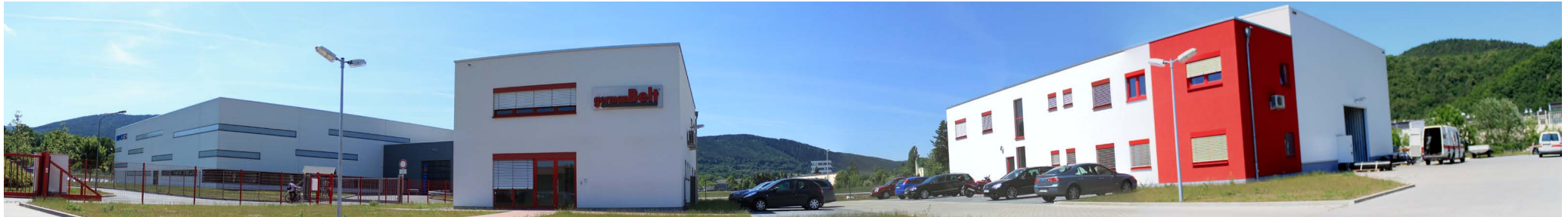
Illustration: Group's headquarter in Bad Blankenburg, Germany
